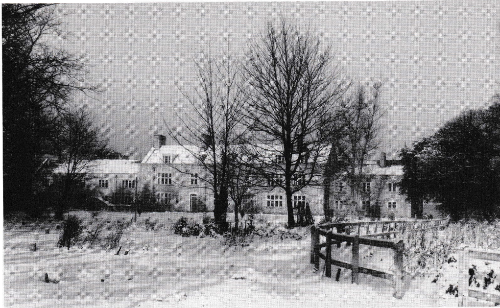
South elevation of Bitterne Manor House after reconstruction as fourteen flats.
